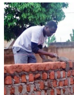
Silver lays some bricks
